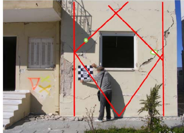
Technology of strengthening the Orthodox churches using the DC90 dampers, the image on the left. Badly damaged building of social housing can be saved by technology of vertical bracing with steel hysteresis shock Absorber System DC90, picture on the right
