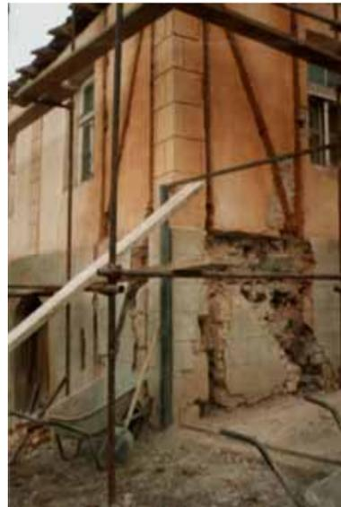
Vertical bracing in considerably damaged stone walls in Jurjevac village.
