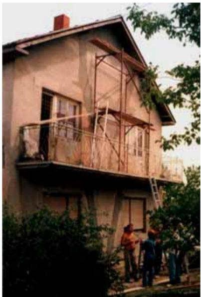
Vertical bracing cemented with fine granulated concrete.
