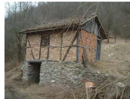
Bondrug system of a water-mill construction in Dobra.
