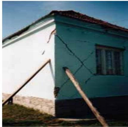
Crossed diagonal cracks on an object in Mionica.
