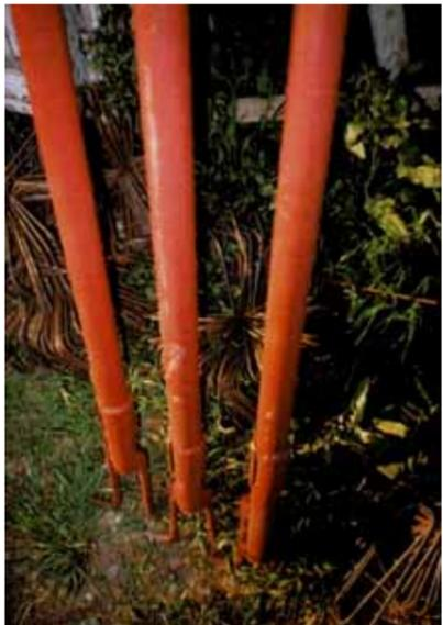
Diagonals with dampers and anchors for strengthening new masonry objects.
