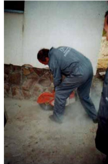
Cutting the sidewalk by diamond saw for digging the foundation collar.
