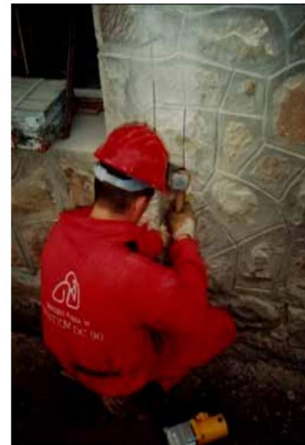
Taking out the stone elements from the wall cut by diamond saw.
