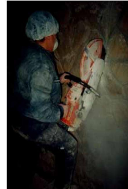
Cutting a stone wall by diamond saw for setting the vertical bracing.
