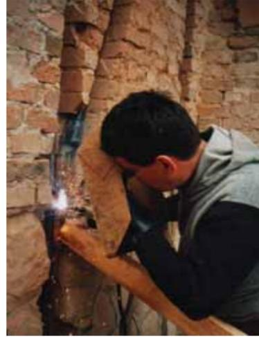
Welding of damper connection with vertical bracing on an experimental object of Lj. Lazic.
