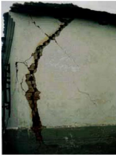
Considerably damaged object with diagonal cracks and wall division.
