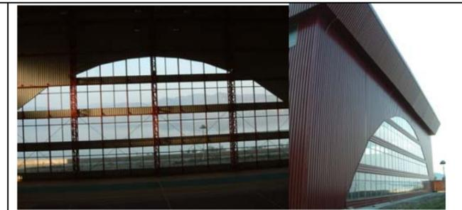
Sports hall in Golubac (42m x 30m x 17m) . Light steel construction in the system of vertical and horizontal bracings-stiffenings on the location IX degrees MCS
