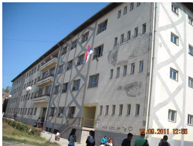
Figure 13. Beginning of retrofit
