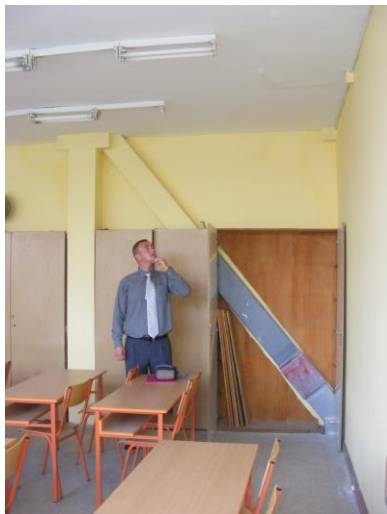
Figure .5. Vertical stiffening in longitudinal Y-direction diagonal square cross-section 260x160x7 with damper. Force in damper +-1100 kN, displacement +-5mm.
