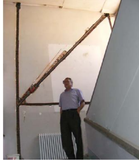
Internal transversal stiffening of the Mechanical engineering school
