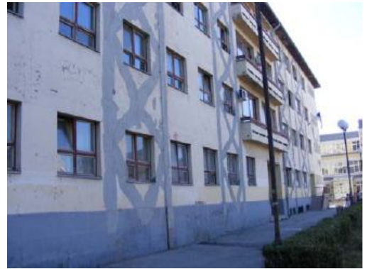
The Facade of the High school
