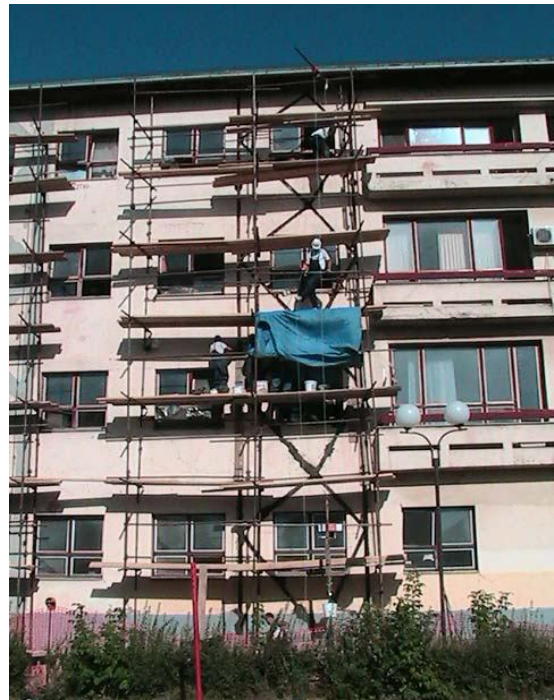
The facade of the Gymnasium (completing bracings with fine granulated mortal)
