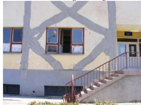
Internal transversal stiffening of the Mechanical engineering school
