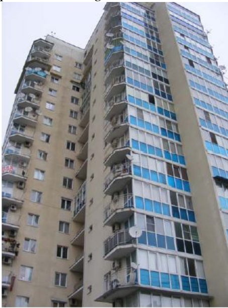
Building P+17 seismically secured by kinematic system in Sochi, Russia 24.09.2011.patent No.200,516 RF and No.1725, ROC), vertical stiffening.
