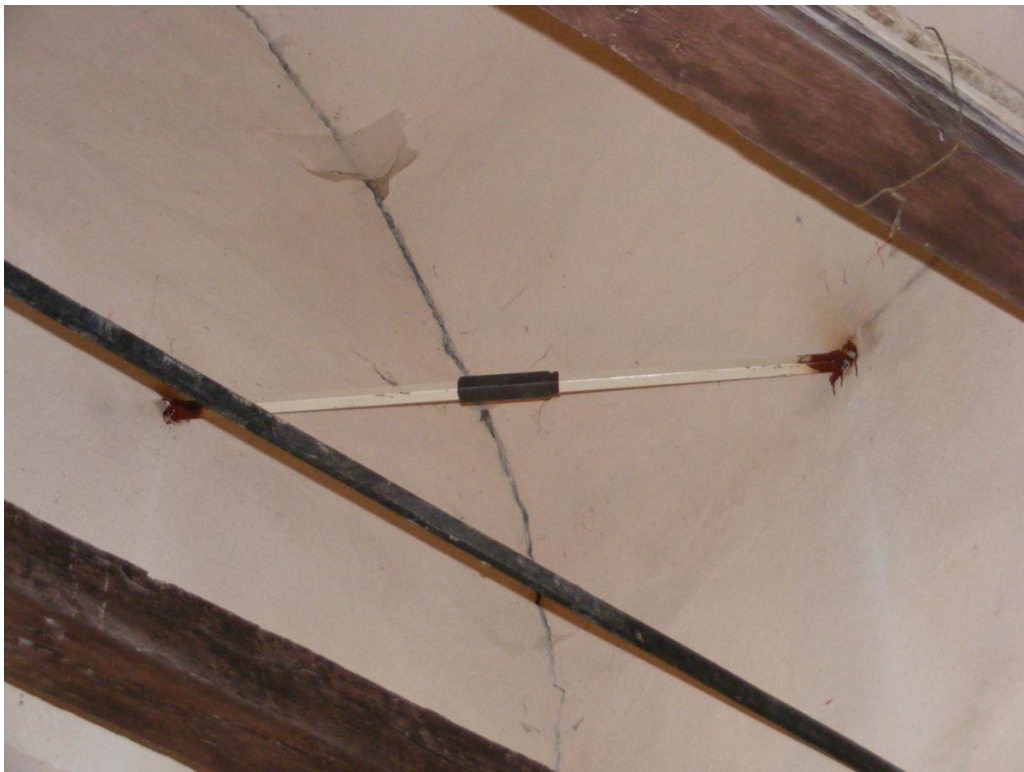
Figure 1. Hysteresis connection transverse wall and façade wall.
