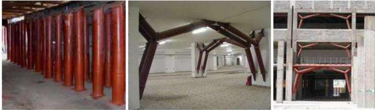
Damper VOGZAL Type - Concrete structure reinforcing
