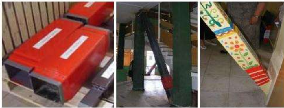
Damper (RHS 260x160x7mm) - Vertical stiffening
