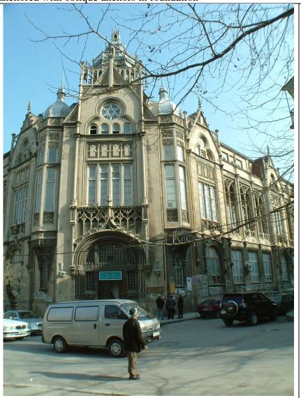
Azerbaijan president residence in Baku is enhanced with thirteen vertical stiffening anchored with oblique anchors in the 120 cm thick massive basic walls. There are applied 66 Dampers of type BAKU and they was built in 11 tons of steel elements (0,1% of whole mass of the object). Object is analyzed on district vibrations and unnatural earthquakes in collaboration with IZIIS Institute from Skoplje, Macedonia
