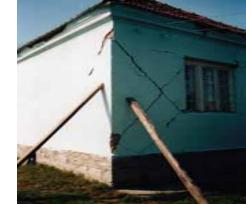
Crossed diagonal cracks on an object in Mionica.
