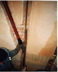
Connection detail of diagonal with damper and vertical bracing, in Lj. Lazich object.
