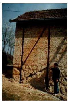
Taking out the stone elements from the wall cut by diamond saw.
