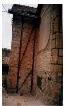
Appearance of vertical bracing, P+1 type, on a house considerably damaged in Lig.
