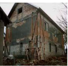
Strengthened object considerably damaged by earthquake and predicted for destruction.
