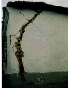
Considerably damaged object with diagonal cracks and wall division.
