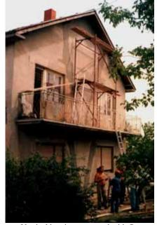
Vertical bracing cemented with fine granulated concrete.
