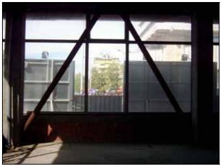
Vertical bracing type"II" for reinforced-concrete or masonry objects.
