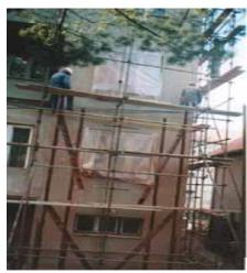
Appearance of vertical bracings type "upside-down P" on four-storey object in Lig.
