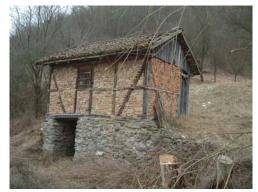
Bondrug system of a water-mill construction in Dobra.
