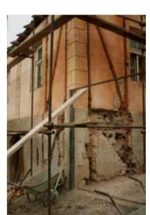
Vertical bracing in considerably damaged stone walls in Jurjevac village.
